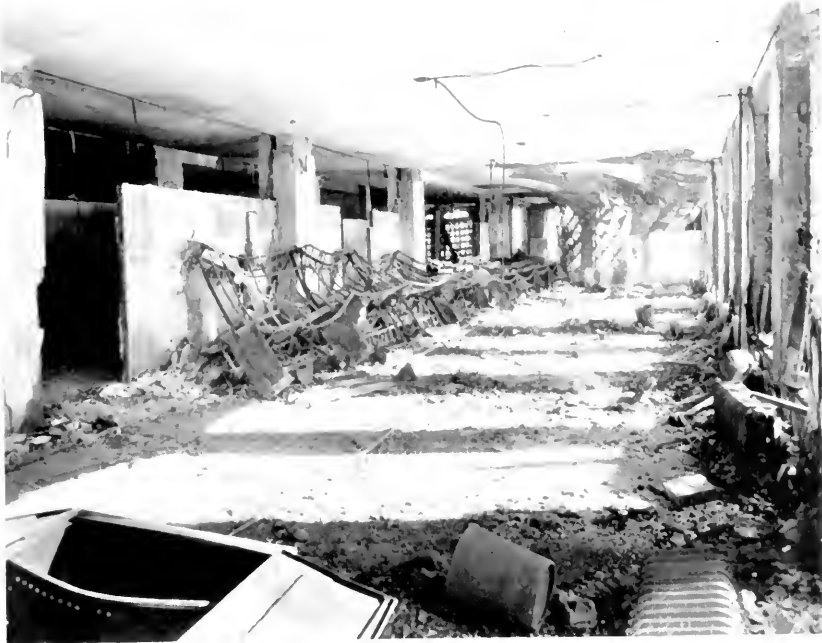
FIGURE 3. WHAT WAS LEFT OF THE LOCAL SWITCHBOARD IN ANDERSON ON THE MORNING OF JANUARY 29.
